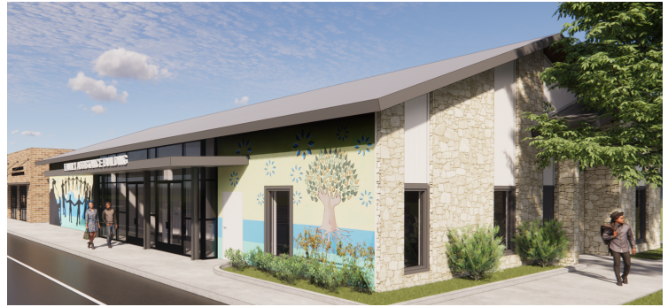
Renovated Family Assistance Center exterior view
